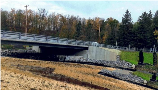
Bridge reconstructed in 2016 heading north towards Deansboro.
