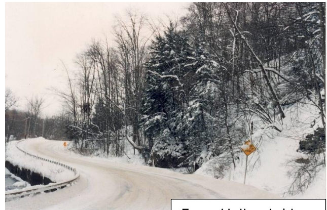
Forge Hollow bridge
